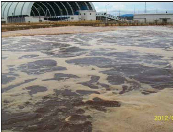
Photo 1. Papermill Wastewater Treatment System
